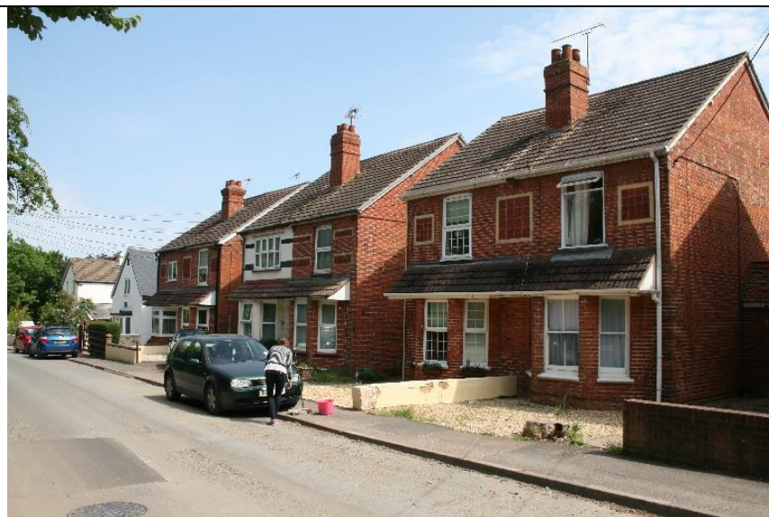
Photo 5. Terraced houses on South View, looking north-east
