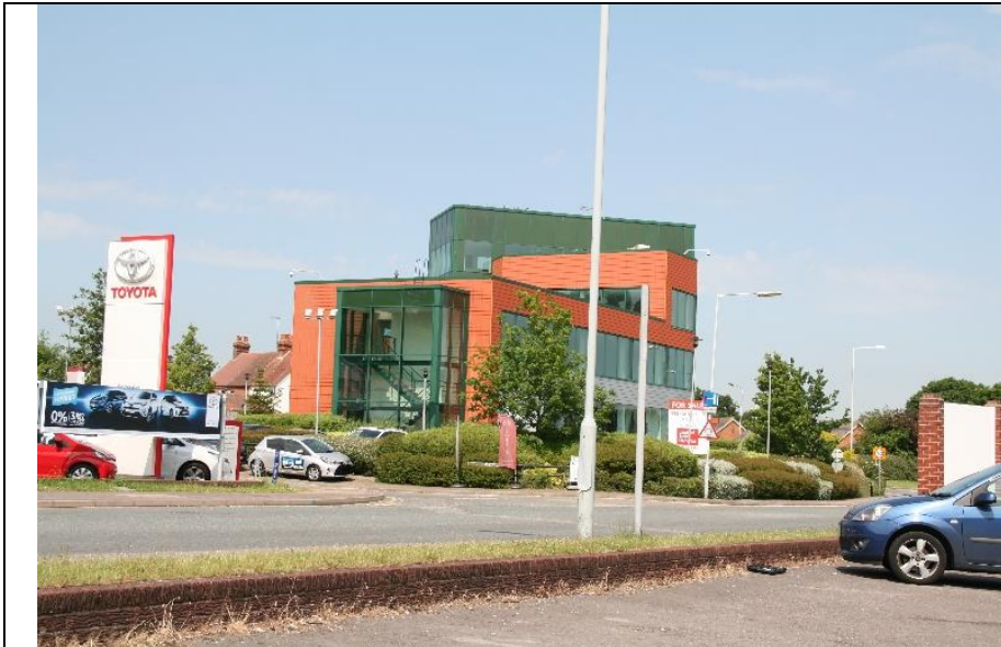
Photo 1. Office block on Cain Road, looking south
