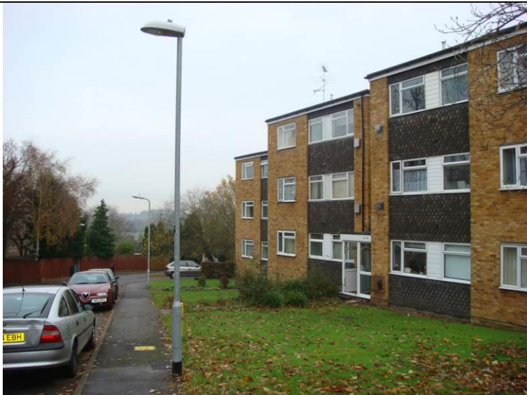
Photo 5. View over Cressex Close Estate to open landscape of PLCA6
