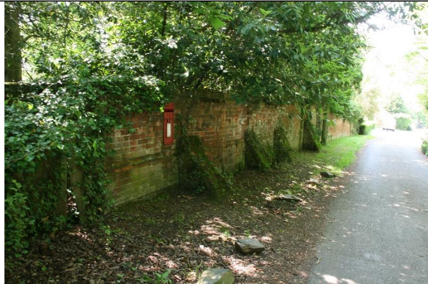
Photo 15. Monks Alley, looking south-west
