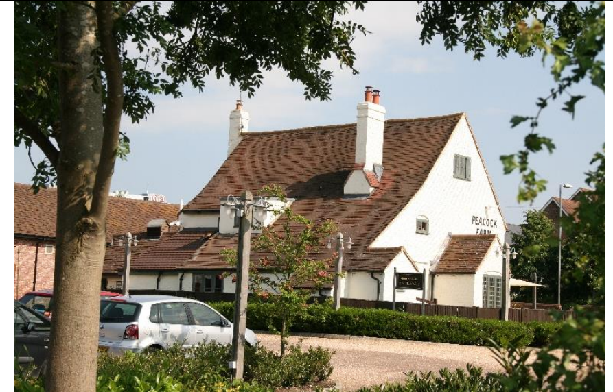
Photo 6. Peacock Farmhouse and outbuildings, looking south-west
