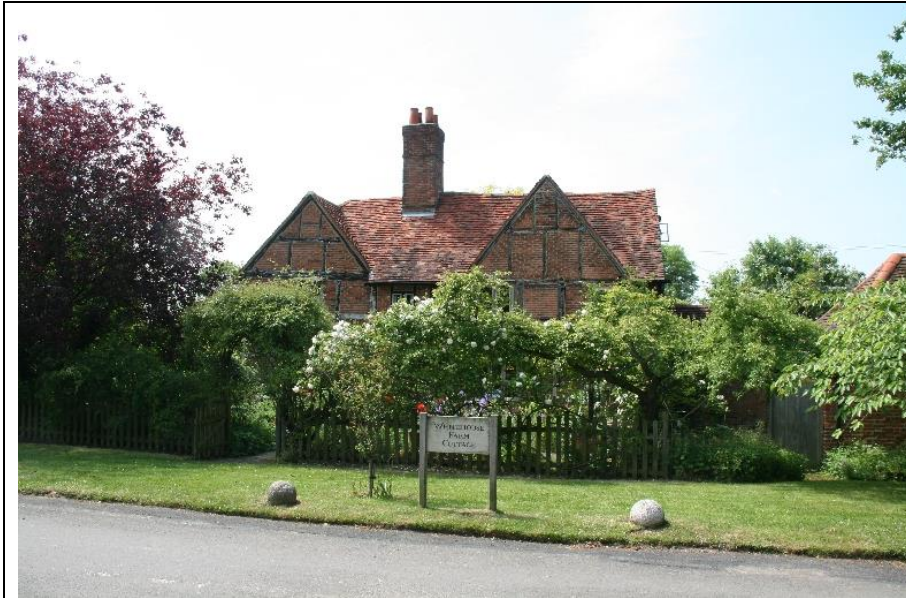
Photo 7. Whitehouse Farm Cottage, looking west
