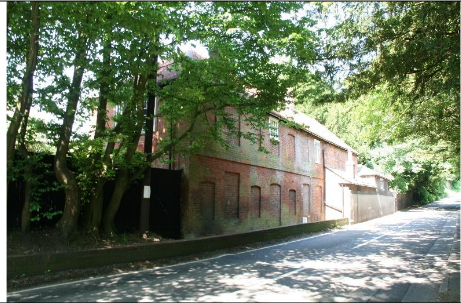
Photo 4. Binfield Court, looking north-west
