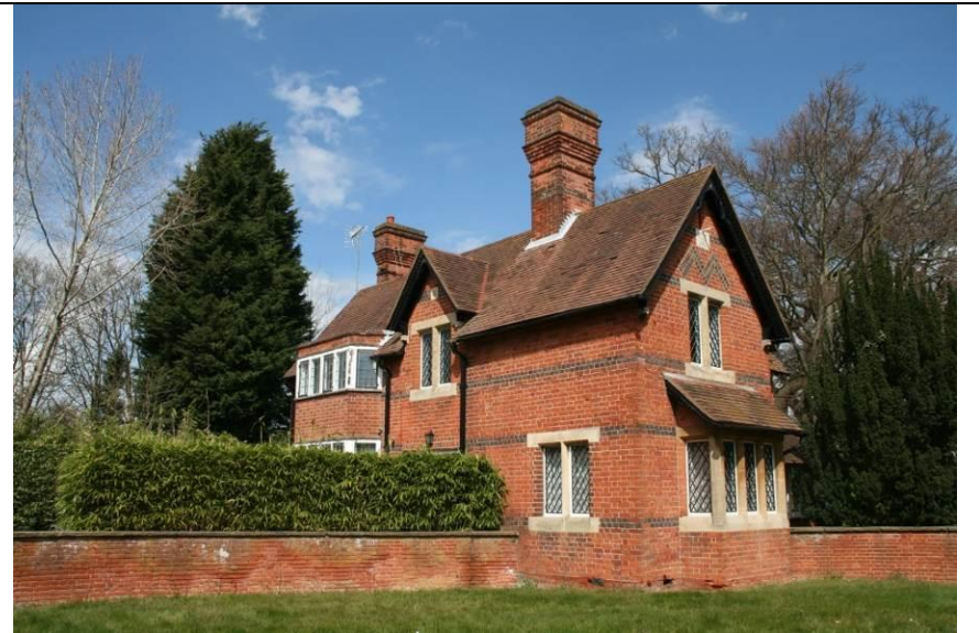
Photo 10: Corner lodge of Newbold College, looking north-east
