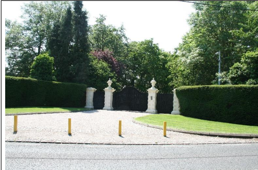
Photo 13. Gates to Binfield Manor on Forest Road, looking south-west
