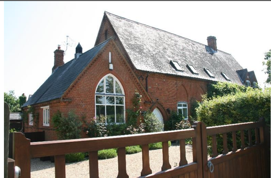
Photo 6. All Saints, former school, looking east
